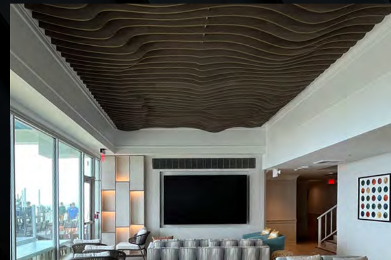
Wood grain printed acoustic baffle in recessed ceiling.
